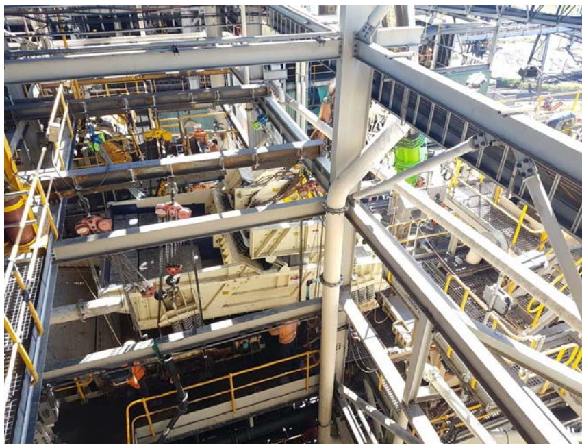
Fig 9 New two mass screen being inserted horizontally into position
